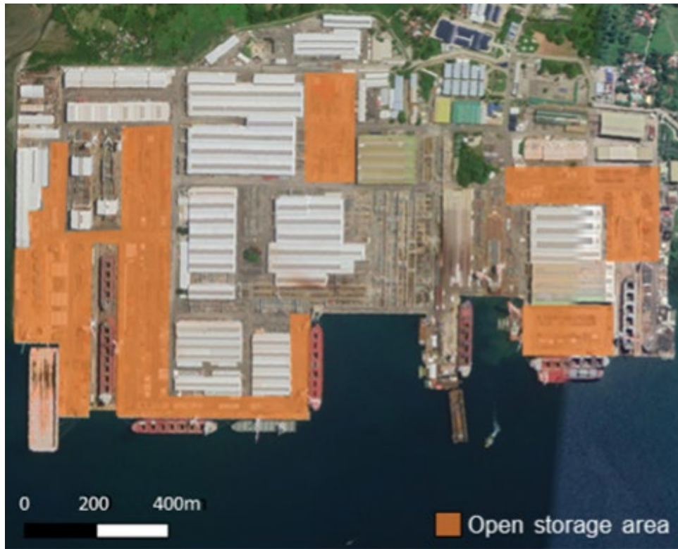
FIGURE 19.7 TSUNEISHI HEAVY INDUSTRIES - BALAMBAN - CEBU
