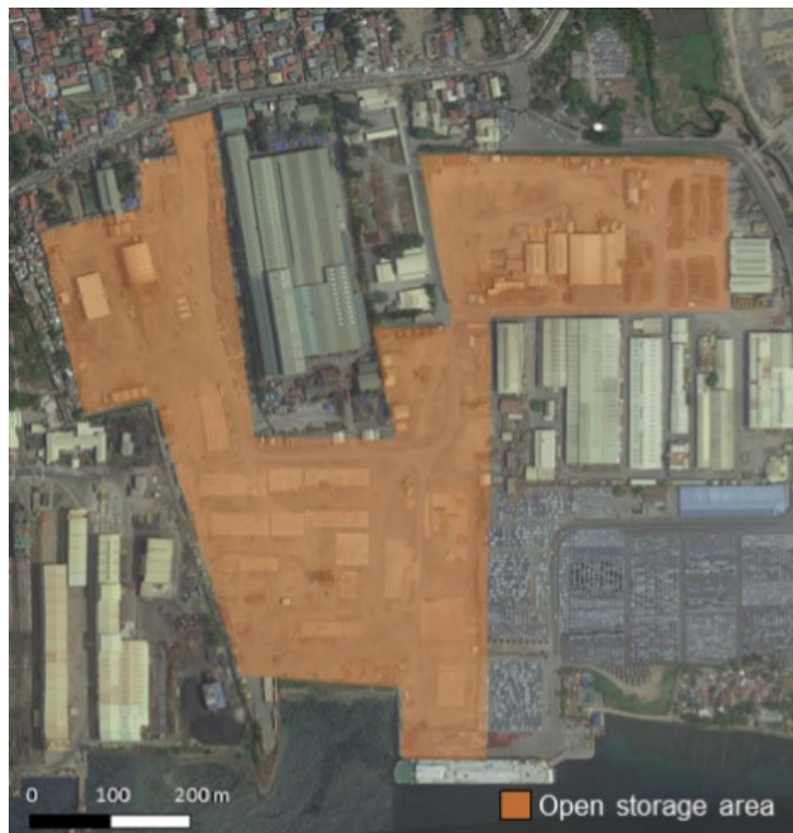
FIGURE 19.3 BATANGAS HEAVY FABRICATION YARD
